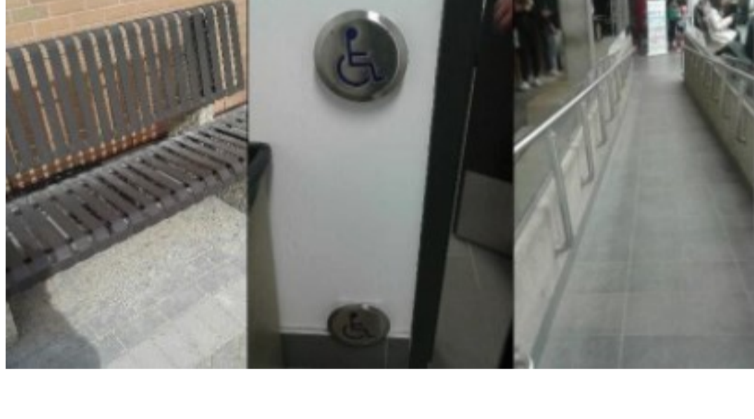
"A bench to sit on now and again is helpful" "Two levels of door opener" "Handrails on either side"
